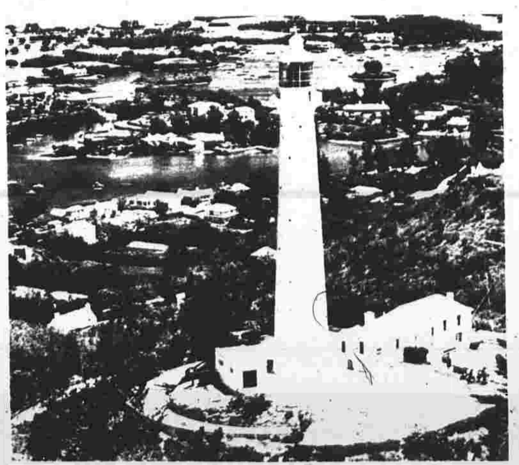
Bermuda's Gibb's Hill Lighthouse is one of the few lighthouses in the world made of cast iron. It stands tall, white and imposing — dominating the scenery at the western end of this 22-square mile island and welcomes more than 35,000 visitors a year to the top to view Bermuda.
